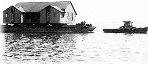
Figure 6: A house being moved from Reedy Island in 1955. The chimneys have been removed from the two extensions at the rear of the house. [11]
