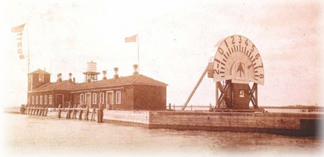
Figure 1: Disinfecting Pier on Reedy Island with the tide indicator in front. [4]
